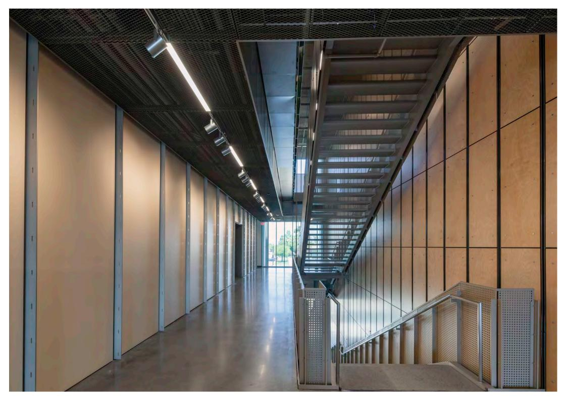
The expanded metal mesh feature ceiling continues outside of the building envelope, and above the main entrances, thereby providing continuity to the architect's design. The external ceilings were designed using a matching aluminum mesh and incorporating requirements specific to an external application such as fixing method and the integration of insect mesh.
