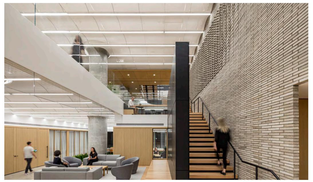
Working closely with project architect, A+I, SAS were called upon to design and supply a custom barrel vaulted ceiling which was installed across six floors of the project. By utilizing micro perforations across the entire face of the panel and employing subtle backlighting, diffused light provides a warm environment contrasting against the striking structural concrete columns.
