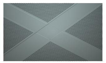
Traditional tartan grid systems make the use of trim strips and crossing boxes suspended from threaded rods and hanger brackets. This detail can be replicated by pressing mock crossing details into the C-Profile. Using C-Profiles instead of crossing boxes provides a far more rigid and durable structure. C-Profiles also provide flexibility to avoid costly bridging around ductwork in the void.
